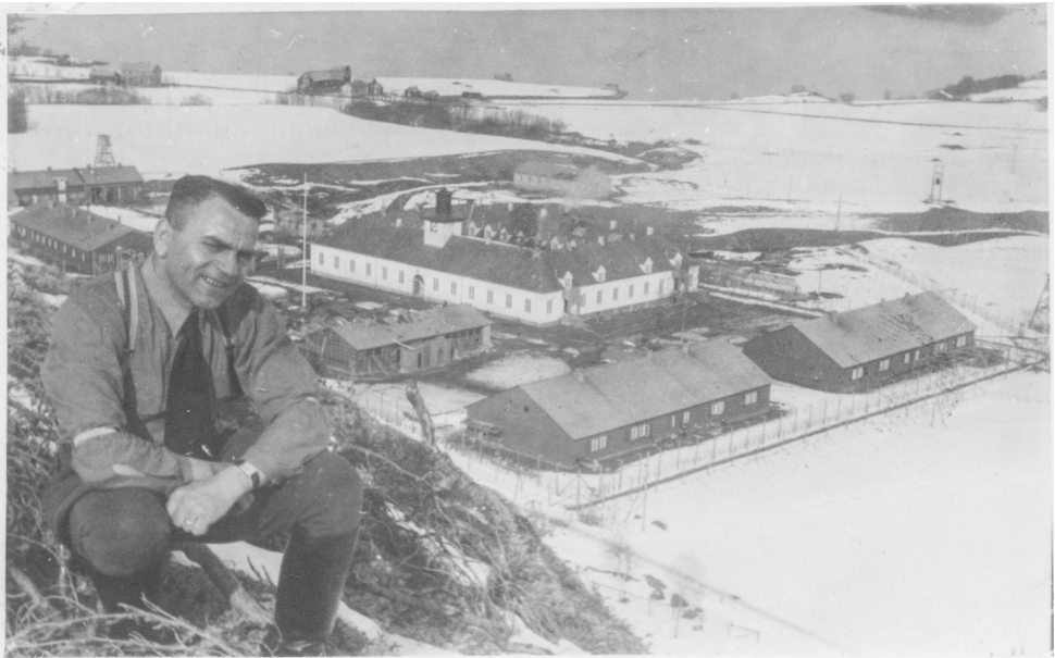
Pic. 11: SS-Strafgefangenenlager Falstad, early in 1944. The sanitary barrack is under construction, the commander's residence (in the background) is newly built. The man in the foreground (German) is unknown. (Falstadsenteret, FSM foto 0800616)
